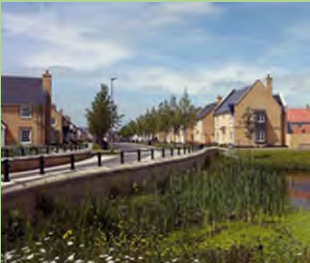
Causeway over brook and attenuation
